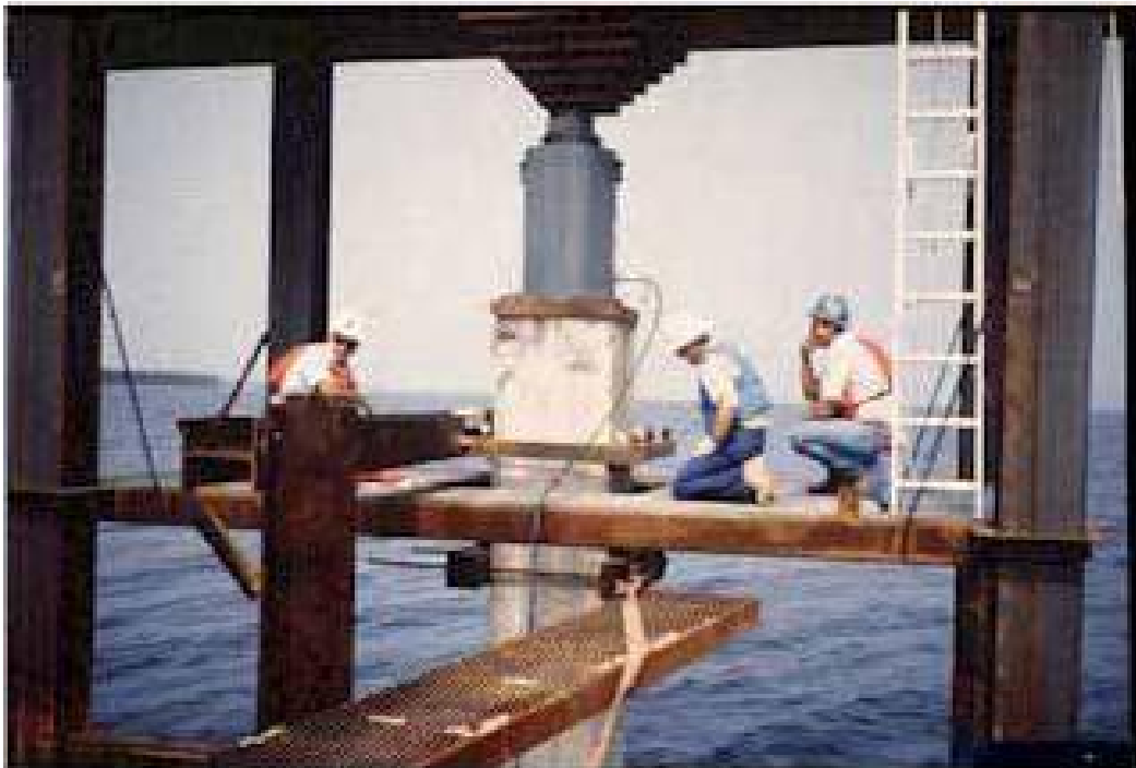
Figure 38, Static Load Test
