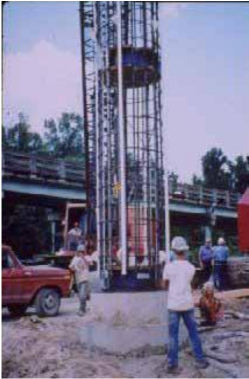
Figure 41, Osterberg Load Cells
