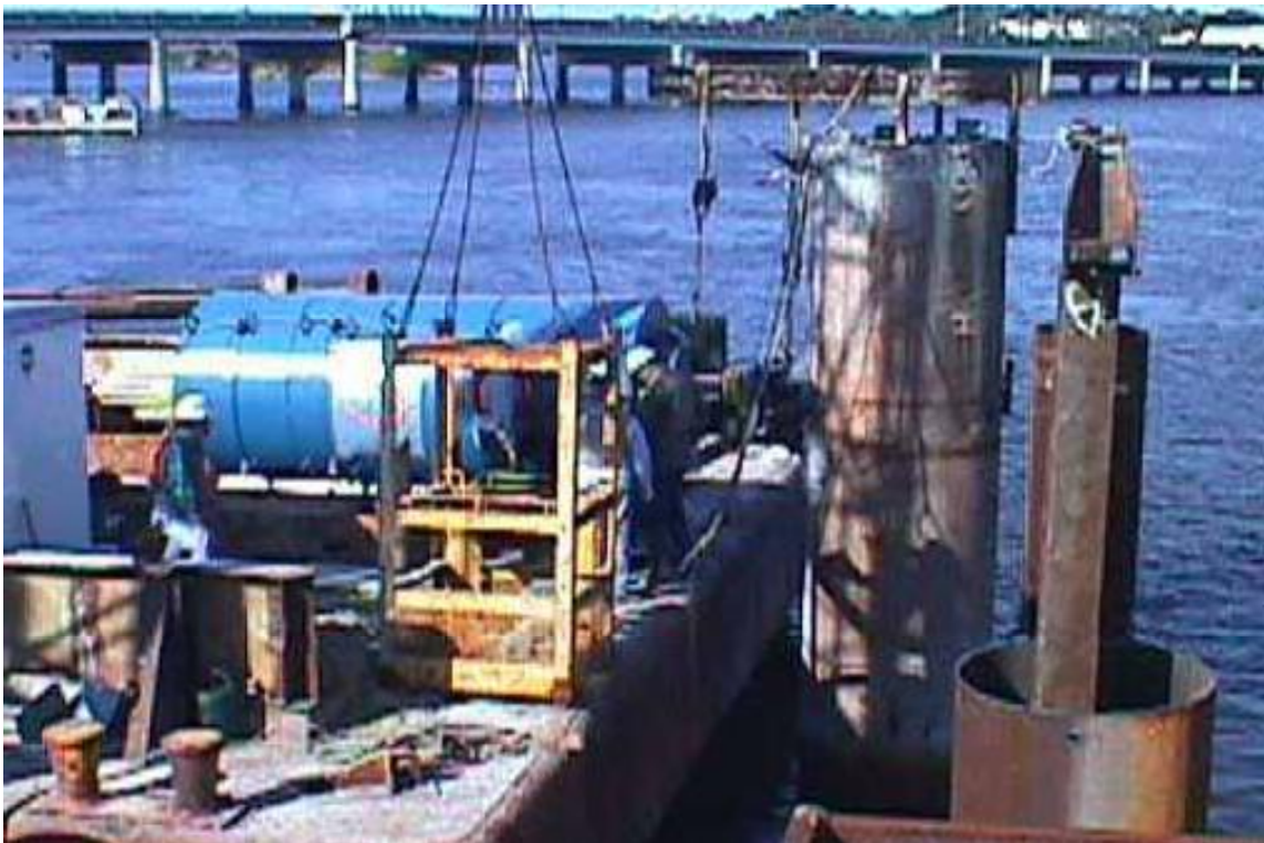
Figure 40, Lateral Statnamic Load Test
