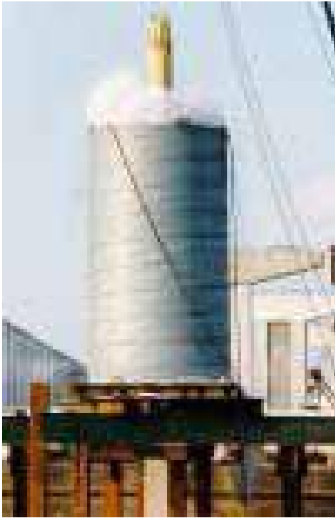
Figure 39, Axial Statnamic Load Test
